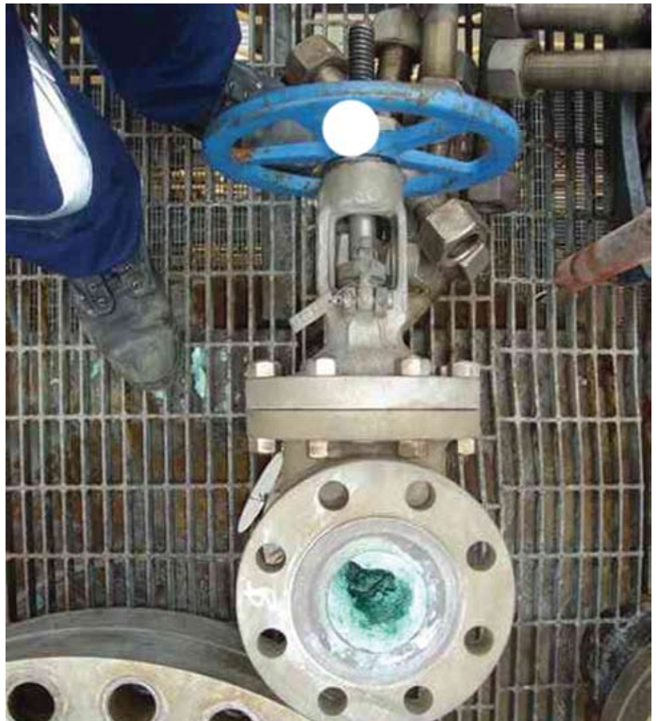
The Class 600LB valve shown top left of the photo replaced 3" and 6" Gate Valves on high pressure, high temperature, acidic, scale forming vapor lines as shown on right.
